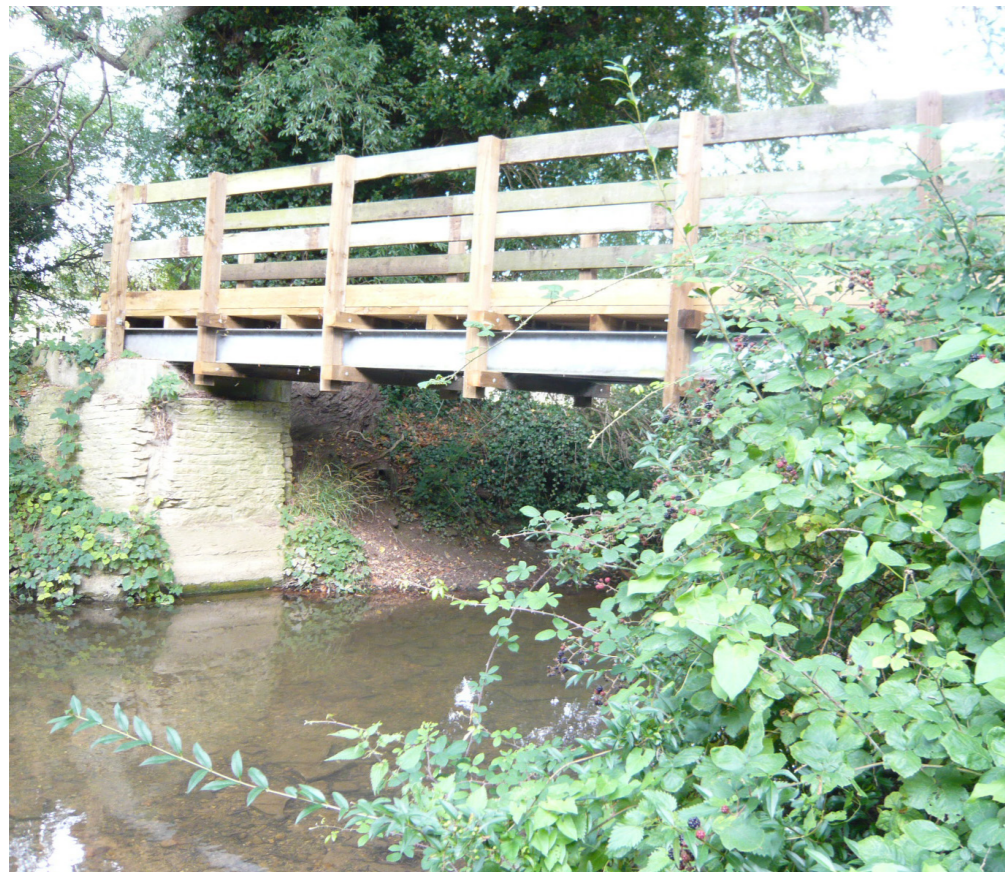
Footbridge over the West Glen River outside of the Order limits.
